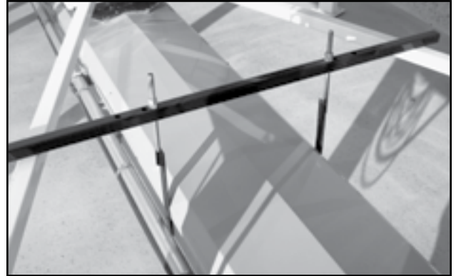
Fig 12 - Hanger bar with brackets bolted on
