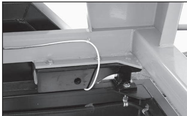
Fig 24 - Load Cells
