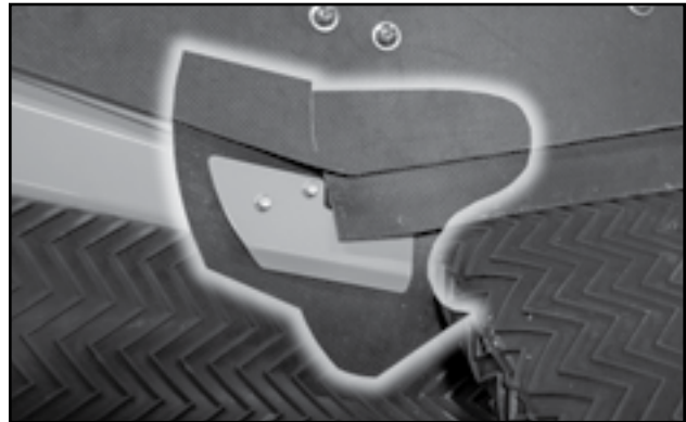
Fig 223 - Flashing clamp holds corner flashing
