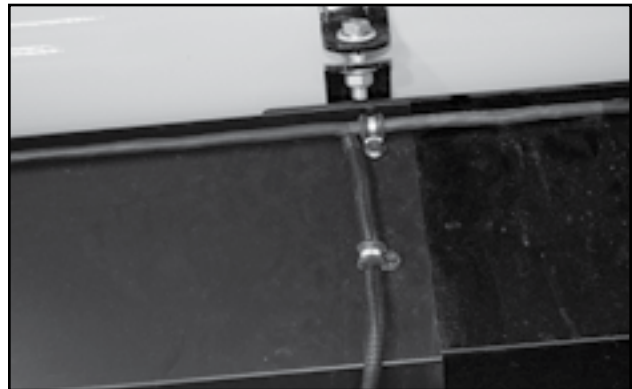
Fig 200 - Anchored wire from light
