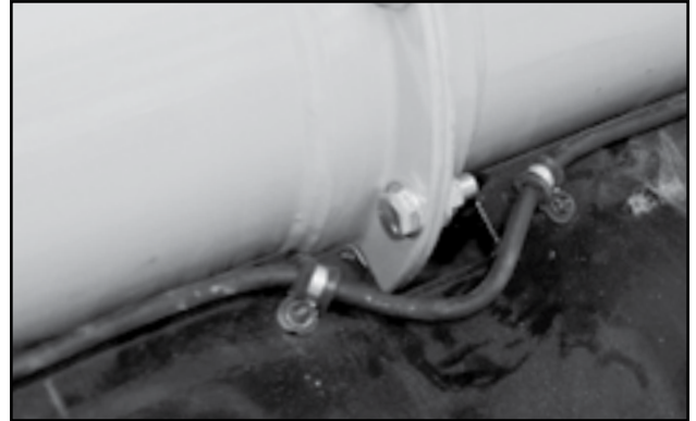
Fig 202 - Wire Around Tube Flange
